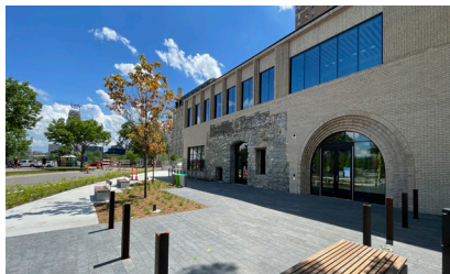
Water Works at Mill Ruins Park
